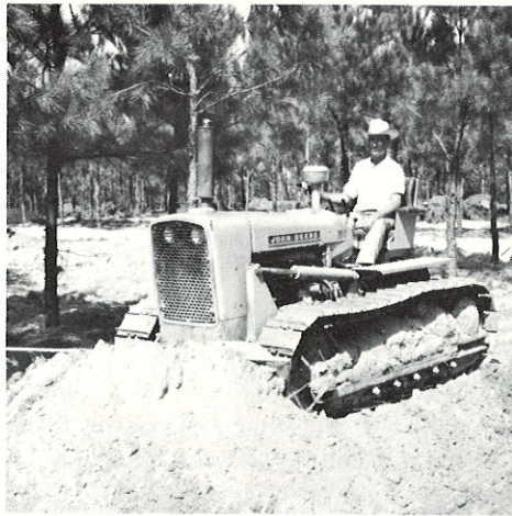
Footpath being leveled by bulldozer. After a layer of coarse red earth is tamped over the path, asphalt paving will be laid providing a 10 foot wide path from the camp grounds to the tabernacle.
